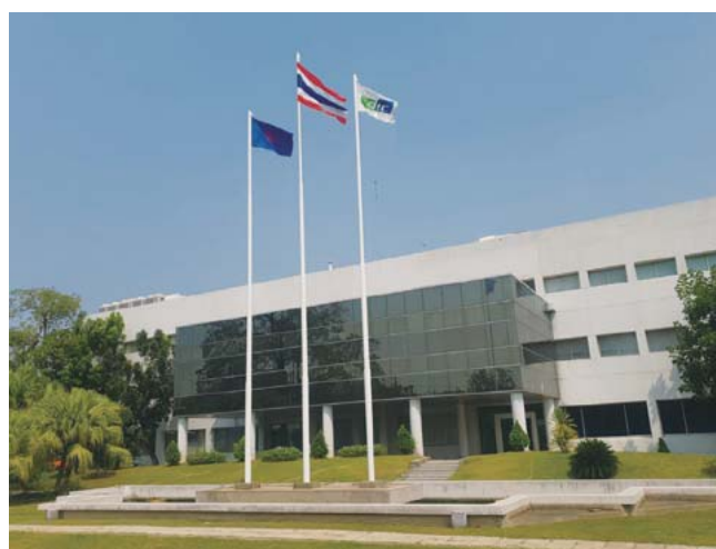
Production facilities for synthetic resins (Thailand)
