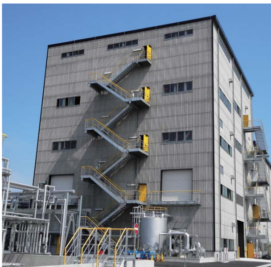
PPS polymer production facility at DIC's Kashima Plant
