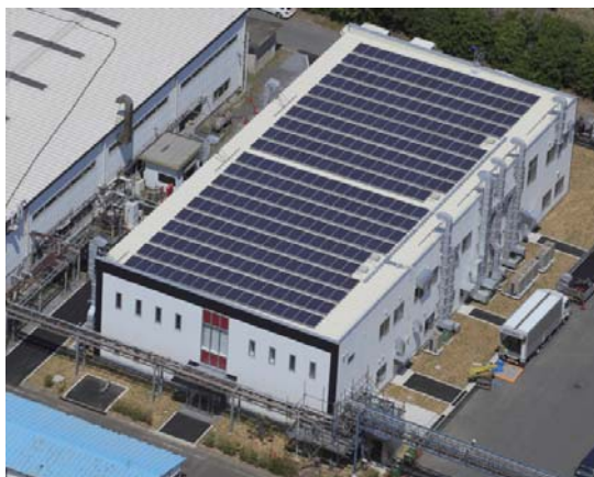
Solar panels installed on the roof of DIC's Kashima Plant
