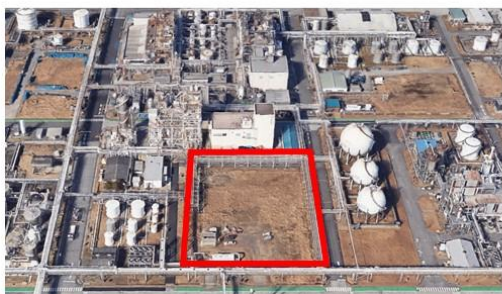
Site of the new production facility at the Chiba Plant
