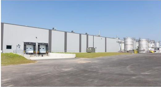
Exterior of Innovation DIC Chimitroniques' new production facility
