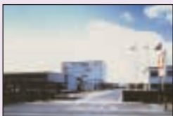
Komaki Plant (Certified under ISO 14001 in March 1998)
