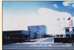
Komaki Plant (Certified under ISO 14001 in March 1998)
