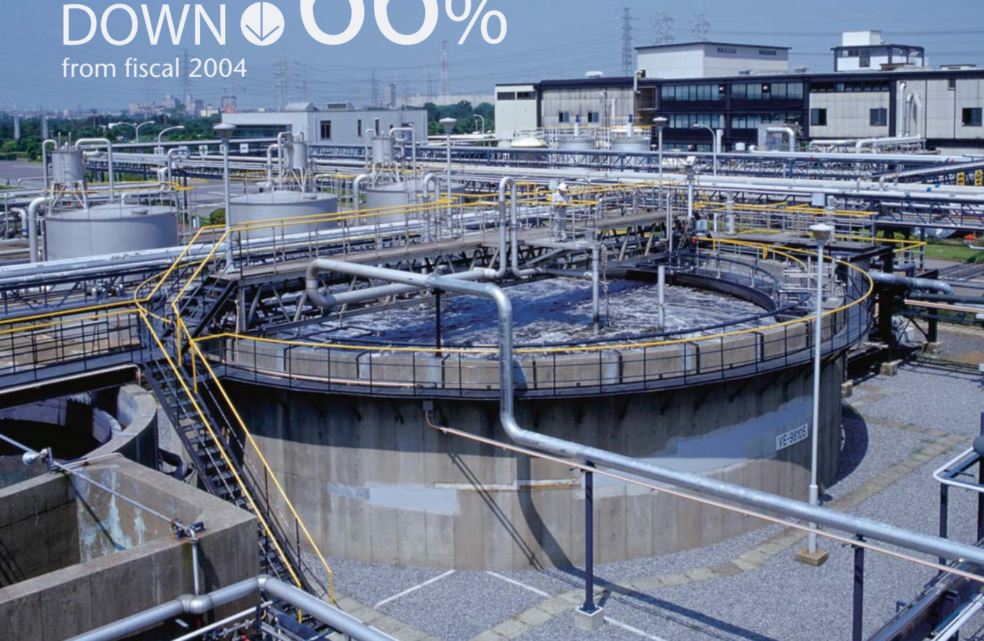
Wastewater processing facility at the Kashima Plant
