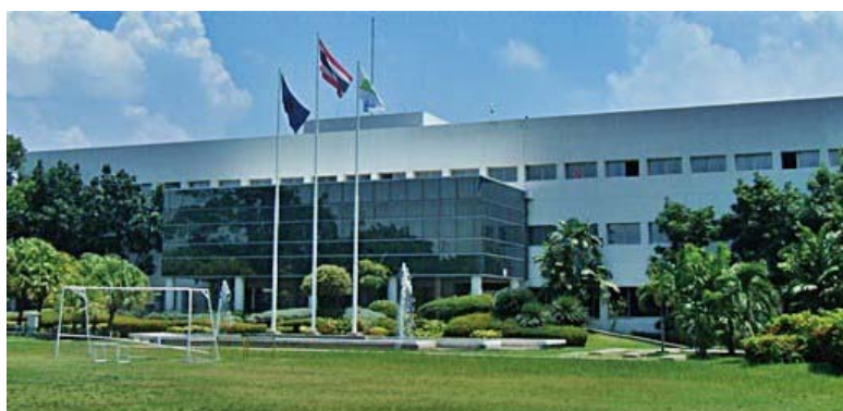
Siam Chemical Industry's plant in Samut Prakan
