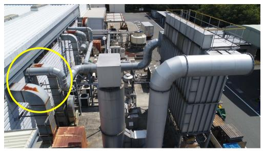
Aerial image captured by a drone confirming the presence of rust on upper section of facility
