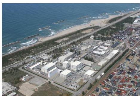
DIC's Hokuriku Plant, which has been fitted with three new multireaction tanks
