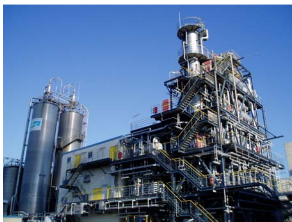
The Yokkaichi Plant's polystyrene production facility
