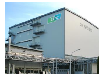
PPS production site, Komaki Plant
