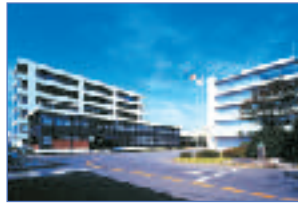
Tokyo Plant (Certified under ISO 14001 in December 1997)
