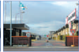
Mikawa Plant (Certified under ISO 14001 in September 1997)
