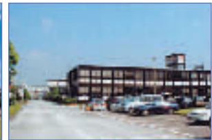
Suita Plant (Certified under ISO 14001 in July 1998)
